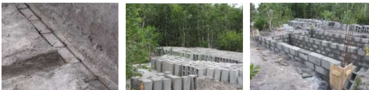
The construction of the first latrine block during Module 1
