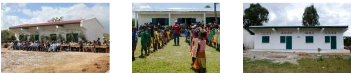
Pictures taken of SEED-built concrete schools at Mahatalaky (left), Tsangoria (centre) and Soanierana (right)
