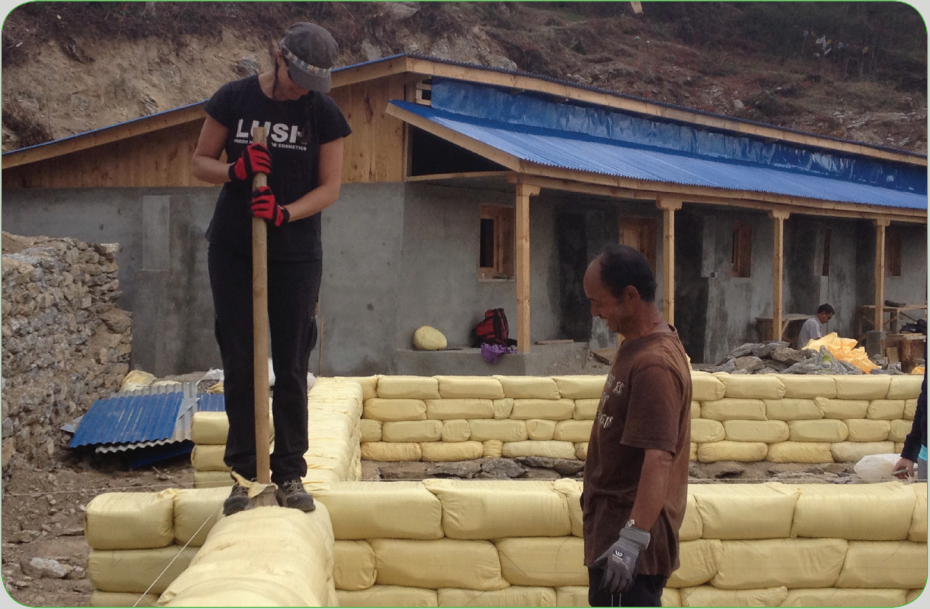
Earthbag Dormitory in Solukhumbu District
