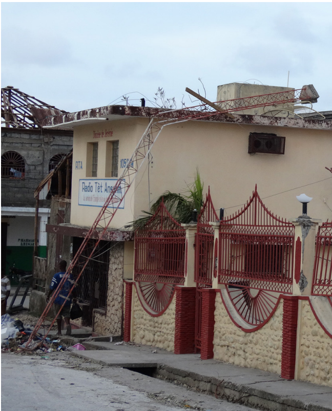
Figure 2 - Toppled antenna
