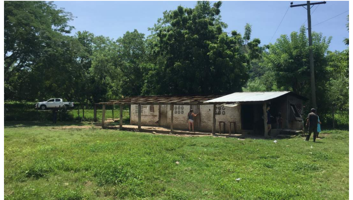
View of the existing structure
