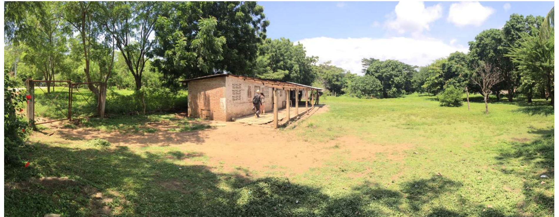
View of the existing structure
