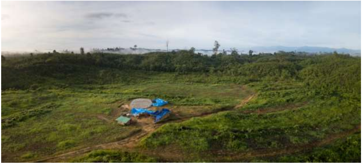
The bamboo school building in progress
