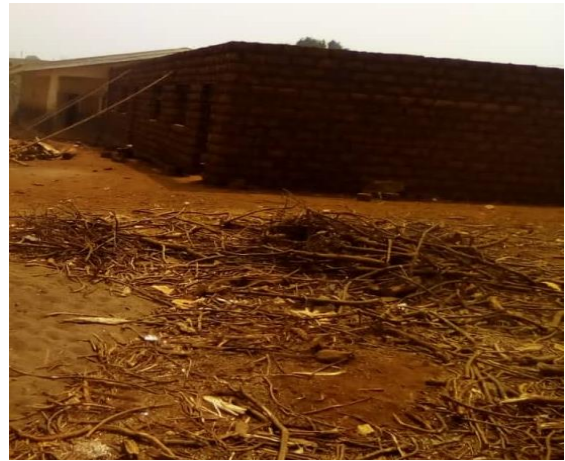
Classroom without a roof
