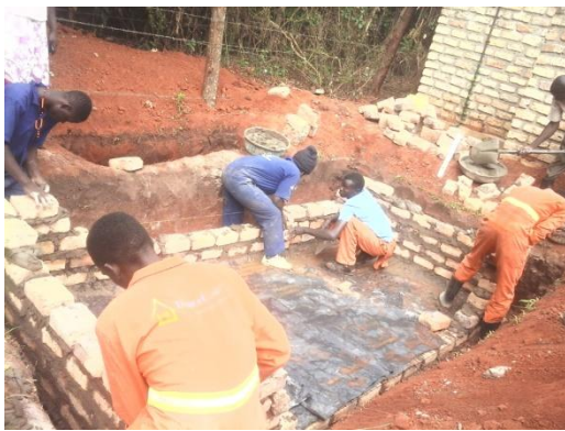
Students of building and cornet practice on the site
