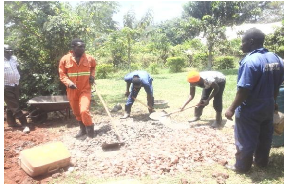
Student of BCP practice how to mix concret
