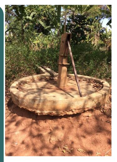
There are few water resources in the rural areas, and a borehole is a priority for clean drinking water. Boreholes range in depth from 30 to 250 feet and are equipped with a simple hand pump. This mechanical pumping system is the most common water delivery method in the Uganda's rural communities.
