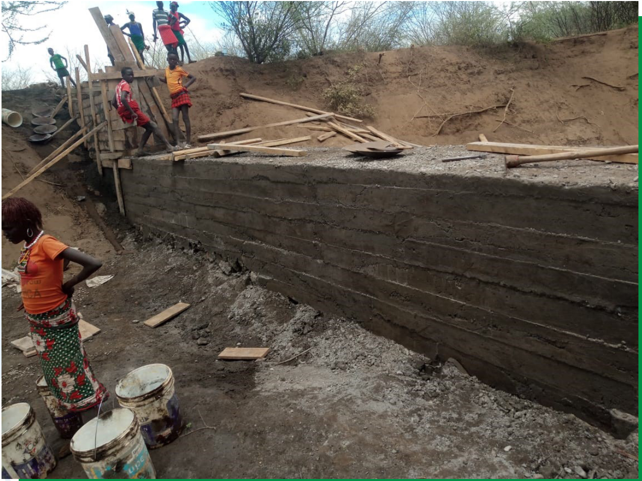
Figure 8: construction and finishing of left and right wings wall
