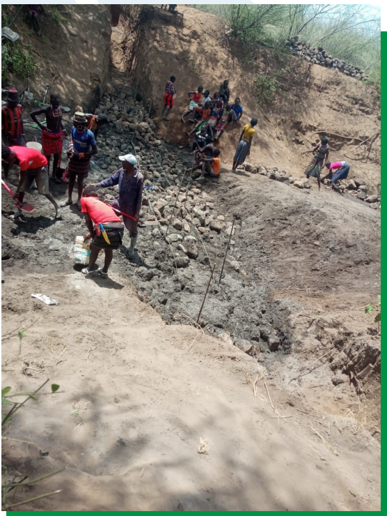
Figure 4: Community members being guided on cement mixing by UDO artisan.
