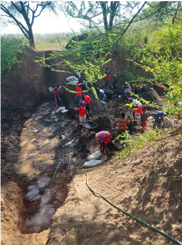
Figure 3: Excavated depth of the trench
