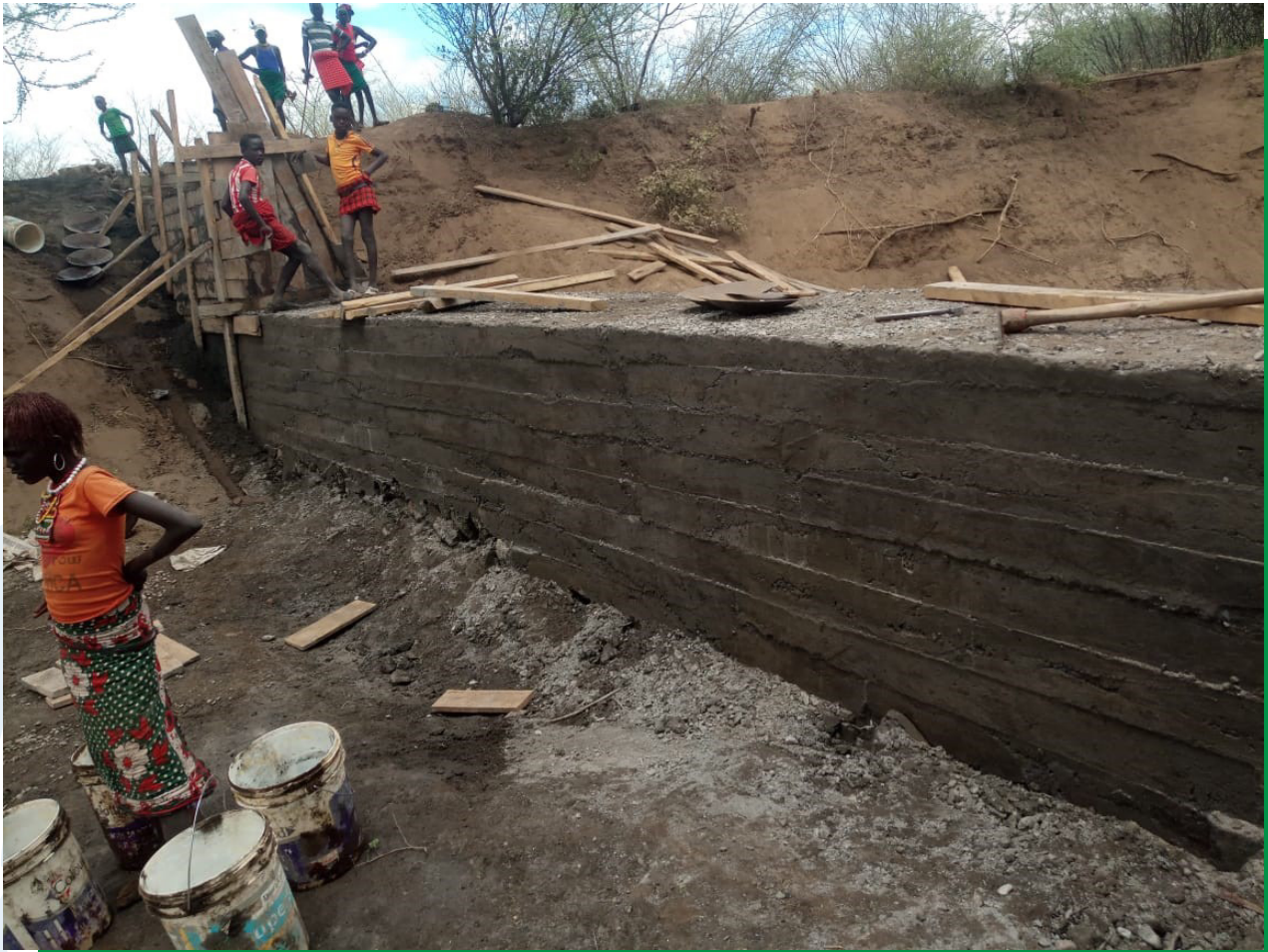
Figure 7: Interlocking of hardcore at 25mm from one to other
