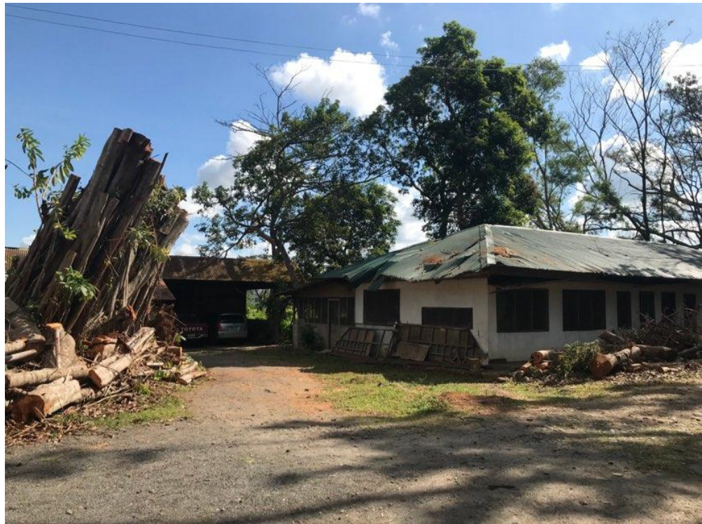
Dormitory and kitchen: After clearing
