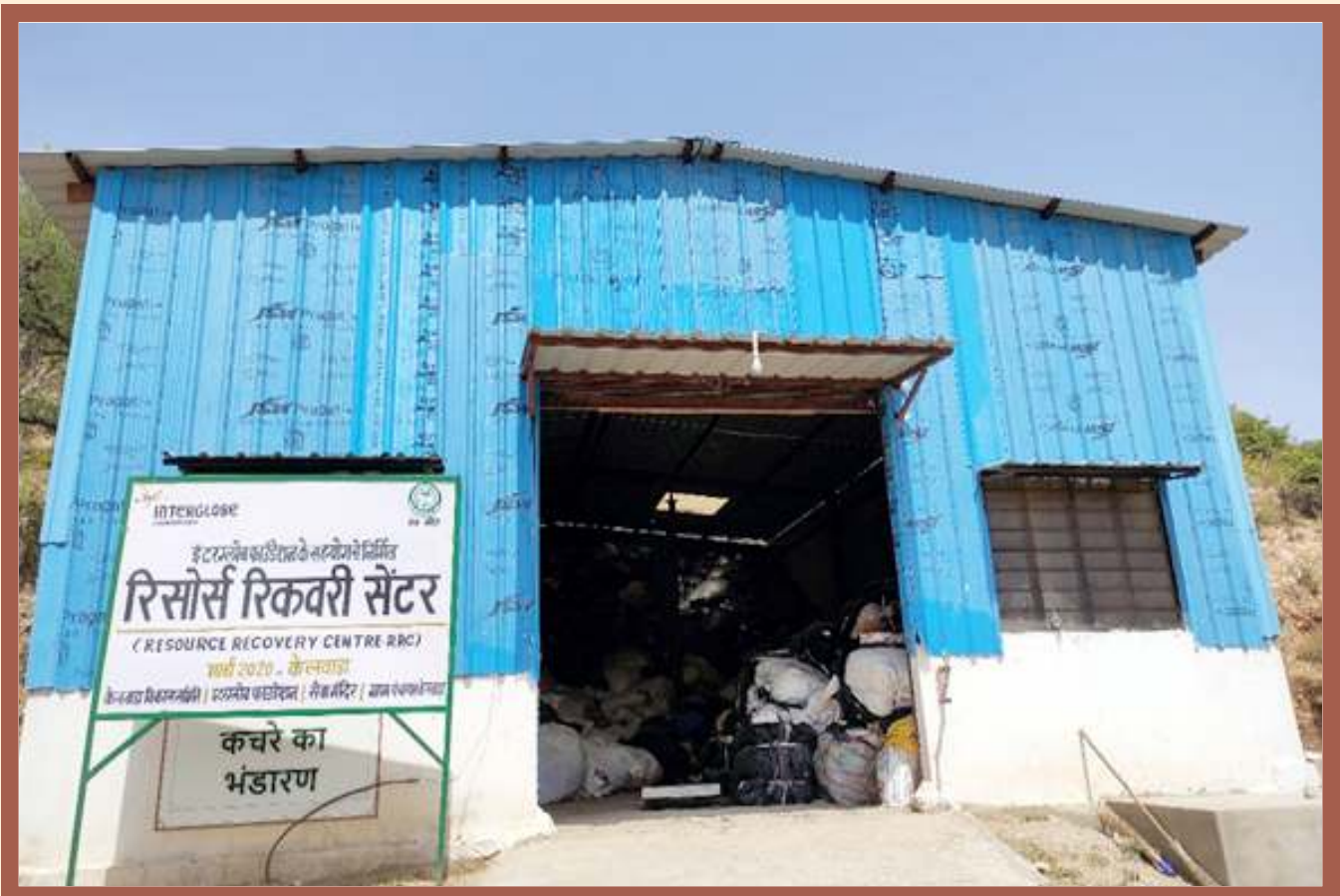
Figure 31: The RRC centre constructed by Seva Mandir through InterGlobe Foundation's support
