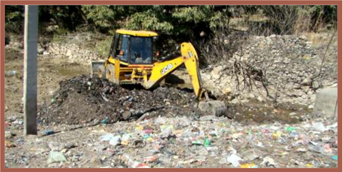
Figure 3: Nearby open plots used as dumping grounds
