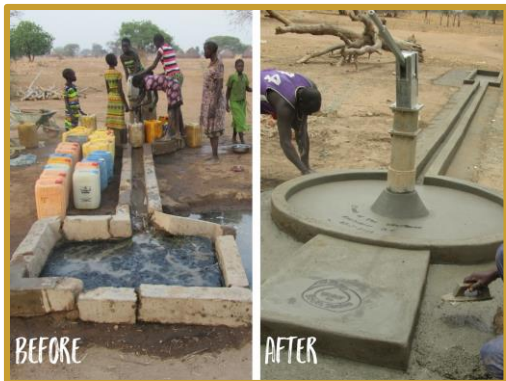
WFSS's new design strengthens the cement platform around the wells.
