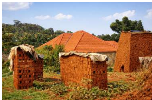
Load-bearing brick masonry base (adobe bricks)
