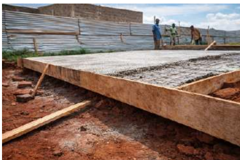
Reinforced concrete foundation
