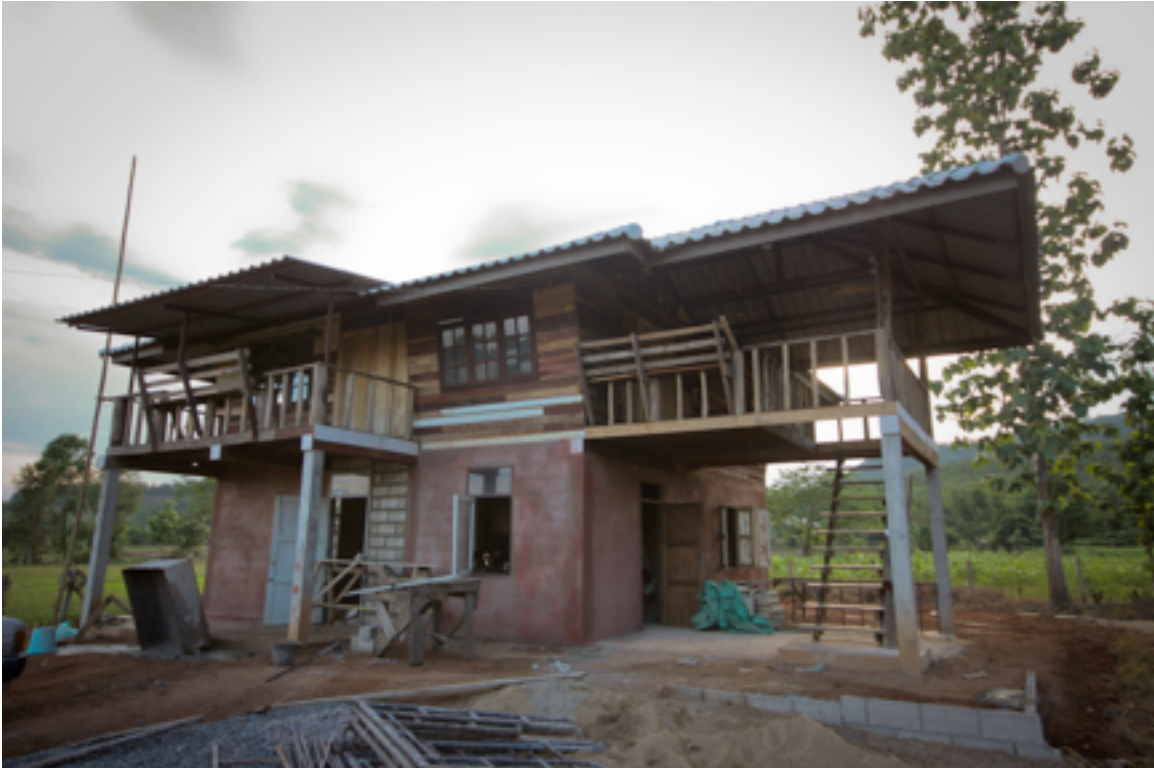
RESOURCE CENTER UNDER CONSTRUCTION / 2010
