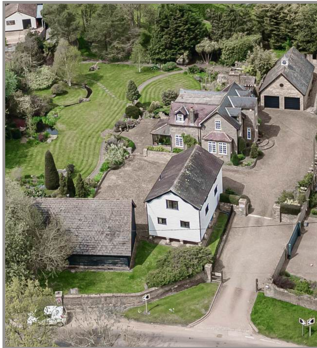
Current view of the site prior to development
