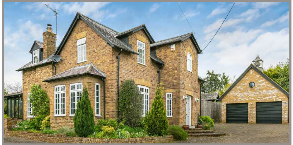
Current existing building
