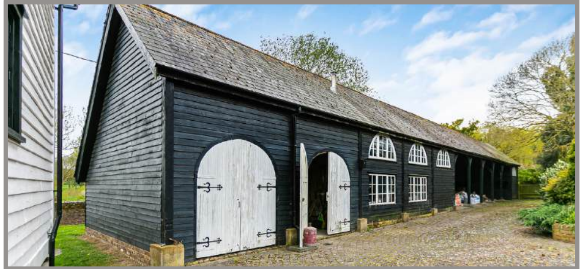
Current existing building
