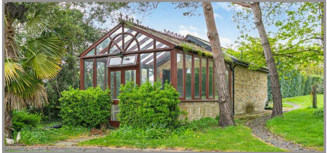
Current existing building
